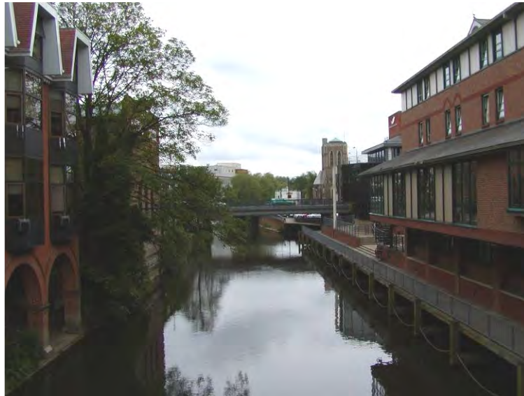
Fig.23 View south from Onslow Bridge
