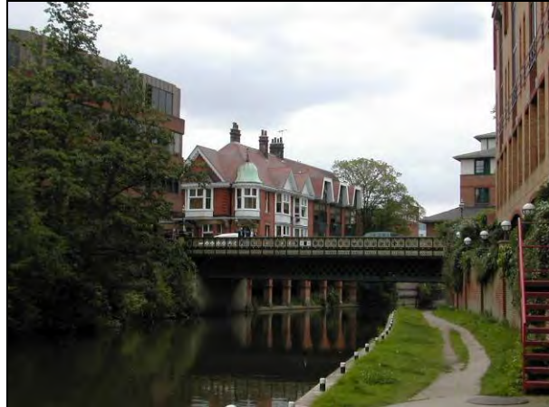
Fig.20 The River Wey, looking south towards Onslow Bridge
