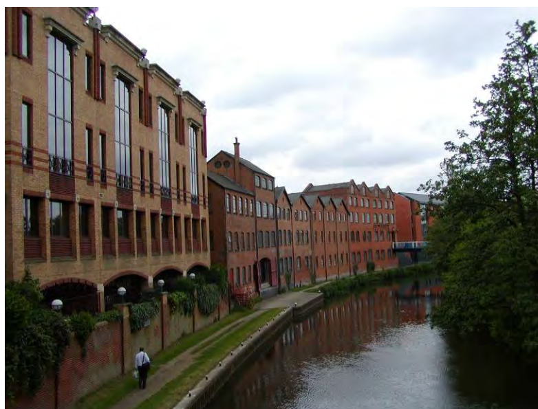
Fig.24 View north from Onslow Bridge
