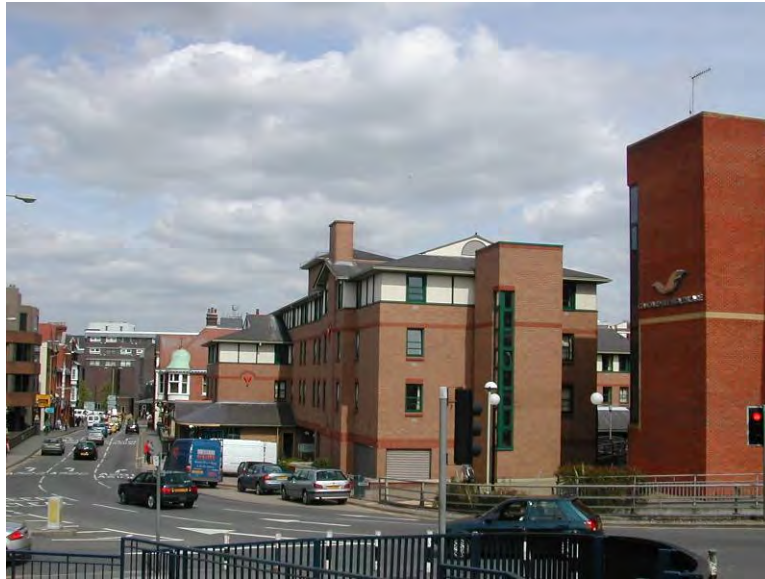
Fig.26 The view down Bridge Street showing the weak YMCA / Wey House corner
