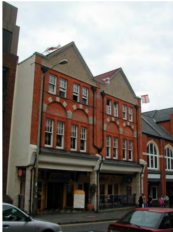
Fig.4 13 and 15 Bridge Street
