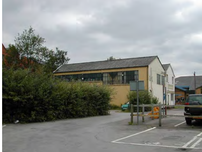
Fig. 13 Weyside Mineral Works, elevation to Bedford Road
