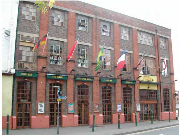
Fig. 8 The Corner House, Bedford Road elevation.
