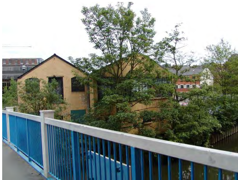
Fig.14 Weyside Mineral Works, riverside elevation
