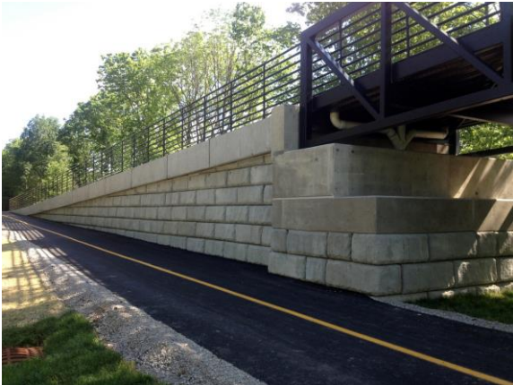
Figure 4: Typical use of Redi-Rock Retaining wall for Bridge Tie-In
