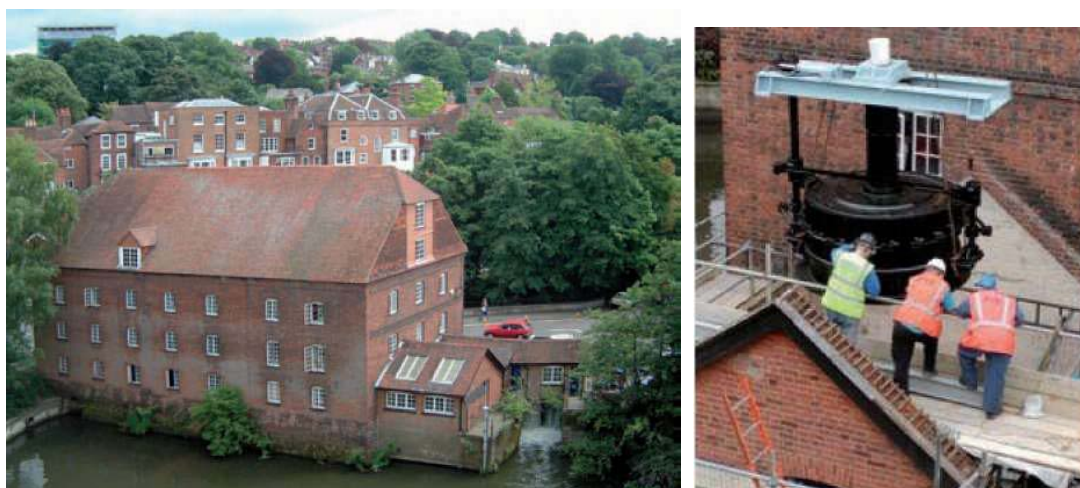
Figure 54: The Town Mill in Guildford showing the single storey Toll House and (right) the 35kW hydro turbine during installation
