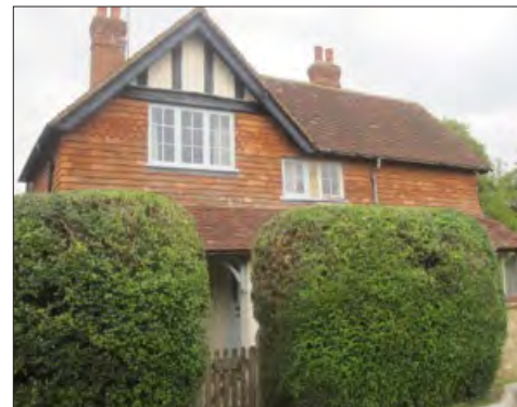
Corner House, Pitland Street
