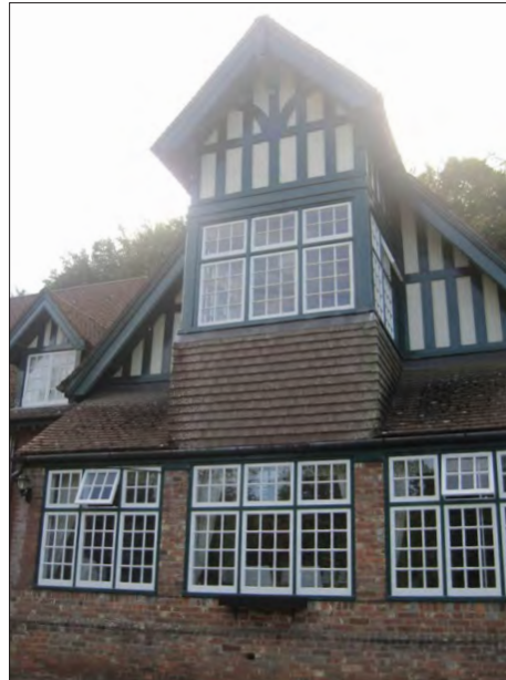
The generous expanse of neo Georgian casement windows to 19th C, Nos. 1 and 2 Lades Court together with 1 and 2 St. Mary's Cottages along the Horsham Road make a striking landmark with its tall, projecting gable, and projecting pentice roof bay at Ground Floor level.
