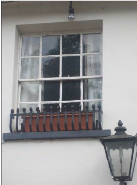
Timber, casement or sliding sash windows, painted white (The Kings Head 18th Circa)
