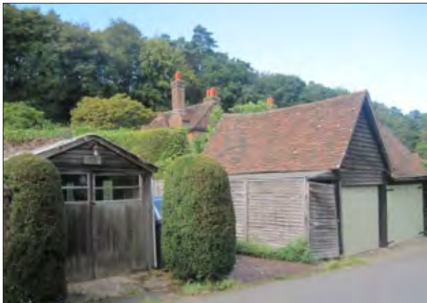
Timber garages to Forest Cottage.
