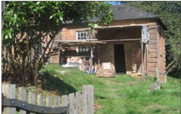
Felday Chapel being restored
