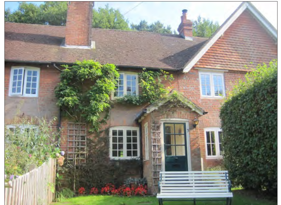
Holmdale Cottages on Felday Glade lane: plain bargeboard with exposed rafter feet; hand made clay tile gable infill, and tall brick chimneys characteristic of Holmbury St. Marys.
