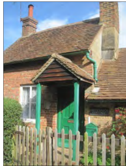
Woodlands Cottage, Pitland Street: tiled, timber clad porch.
