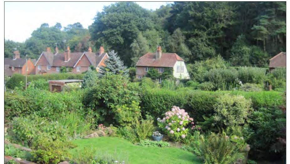
Birdlands and Hurst Cottages; Holmdale Cottages, centre; right, No.4 Felday Glade
