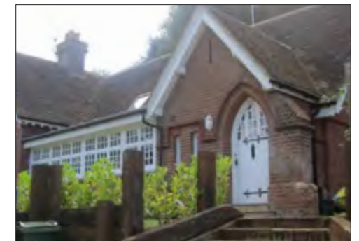
Arts and Craft detailing: Entry porch and Gothic arched door with strap hinges. This steep site is shown by the rising land and many entrance steps.
