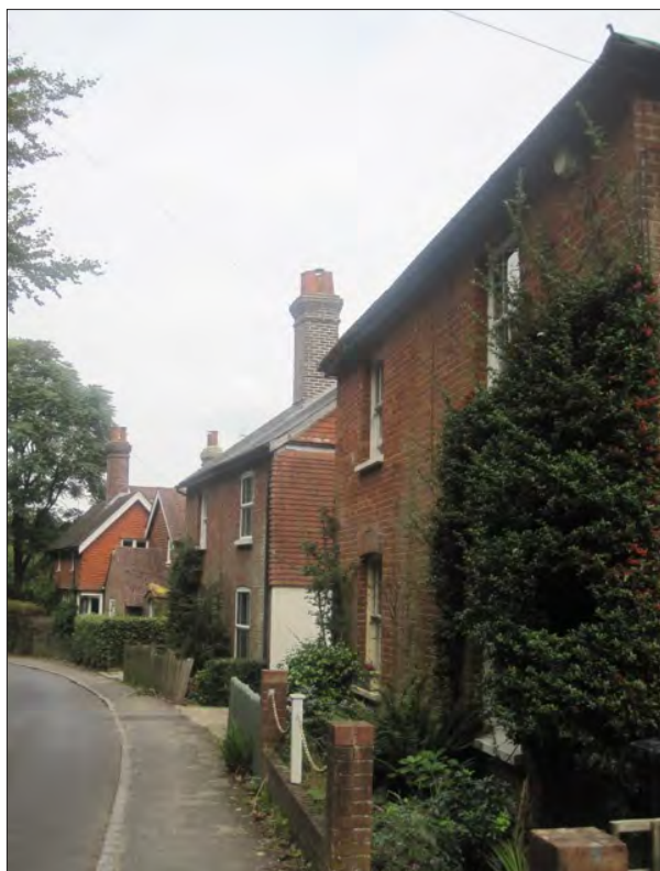
View down the Horsham Road of early Victorian era of 1 to 4 Albion Cottages and Stagbury House, beyond to the north. The prominent chimney stacks, red brick cladding and vertical hanging tiles are typical features.
