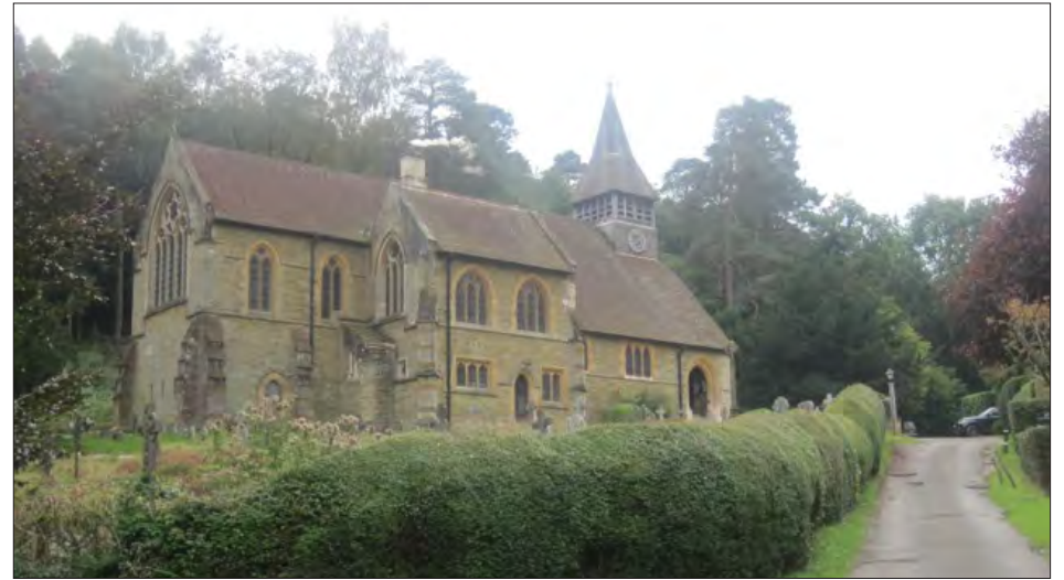
Long view of St. Mary's from Horsham Road, framed by mature hedges.
