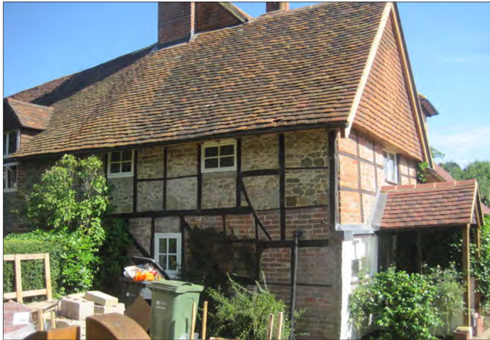
Chapel Cottage, a Grade II Listed Building.
