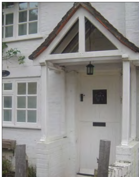
Porch at Rose Cottage with typical plain clay tiled roof, swept eaves and open framed gable end.
