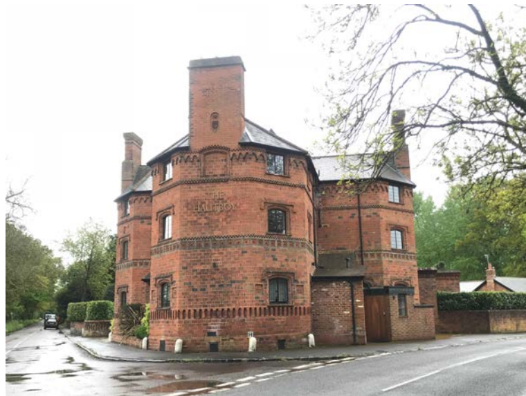
Figure 18: The former Hautboy Inn, Ockham Lane and Alms Heath
