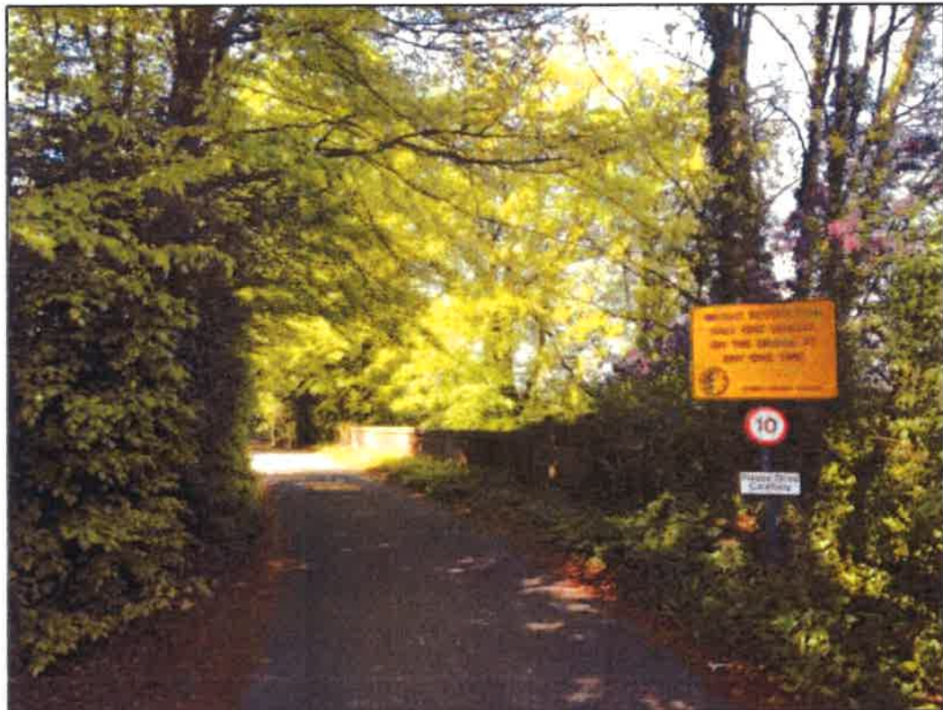
Figure 1 – Down Place at A3 northbound on-slip overbridge
