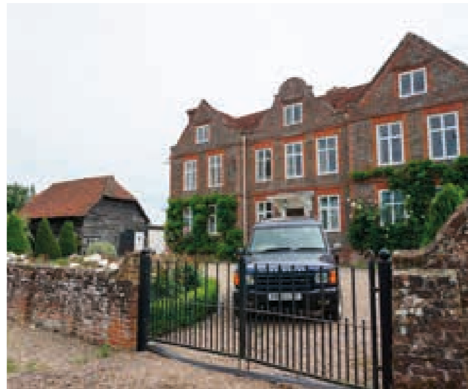
Listed Littlefield Manor and barn (from the west)
