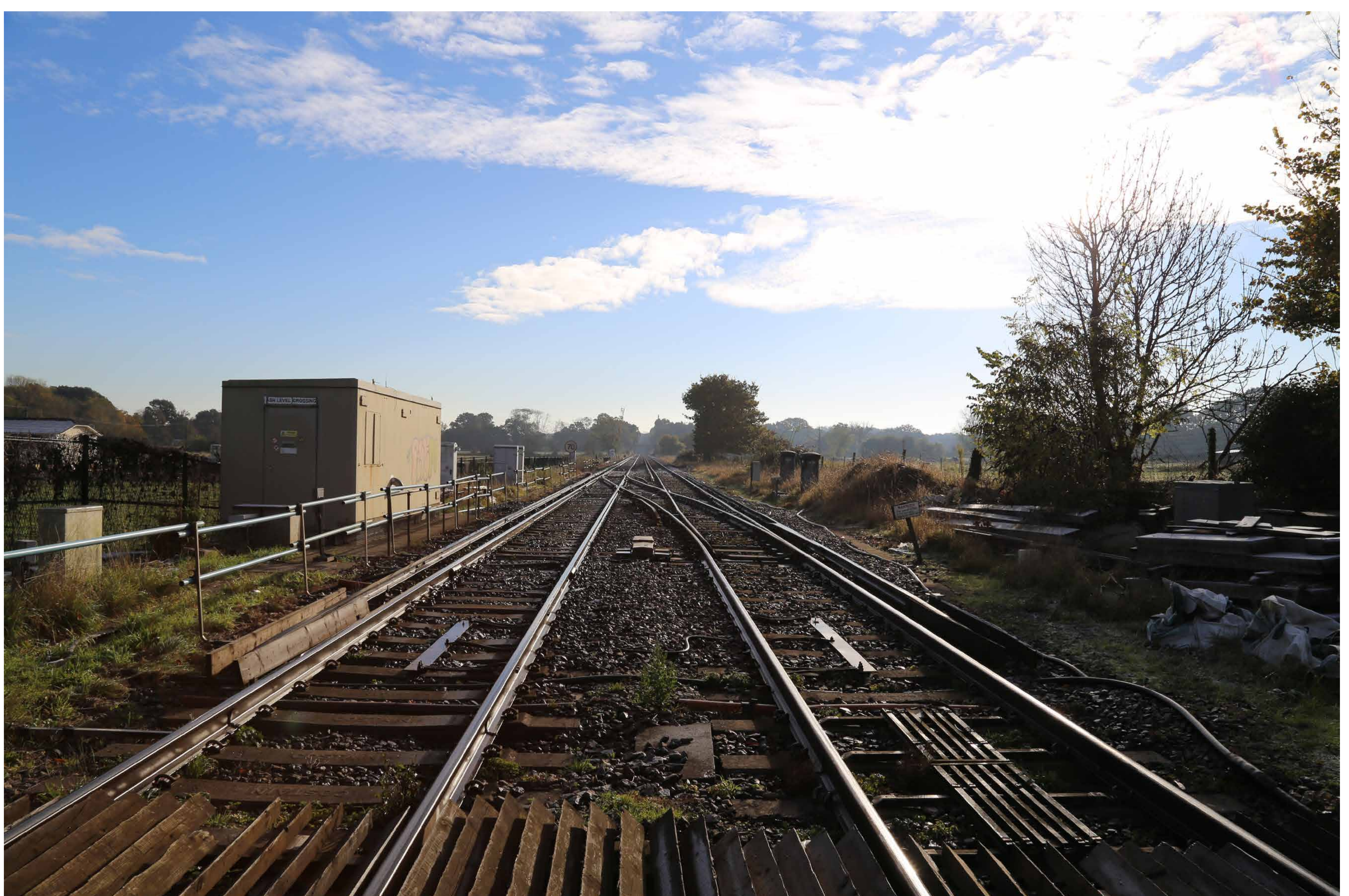
North Downs Line (Ash Level Crossing looking south east)
