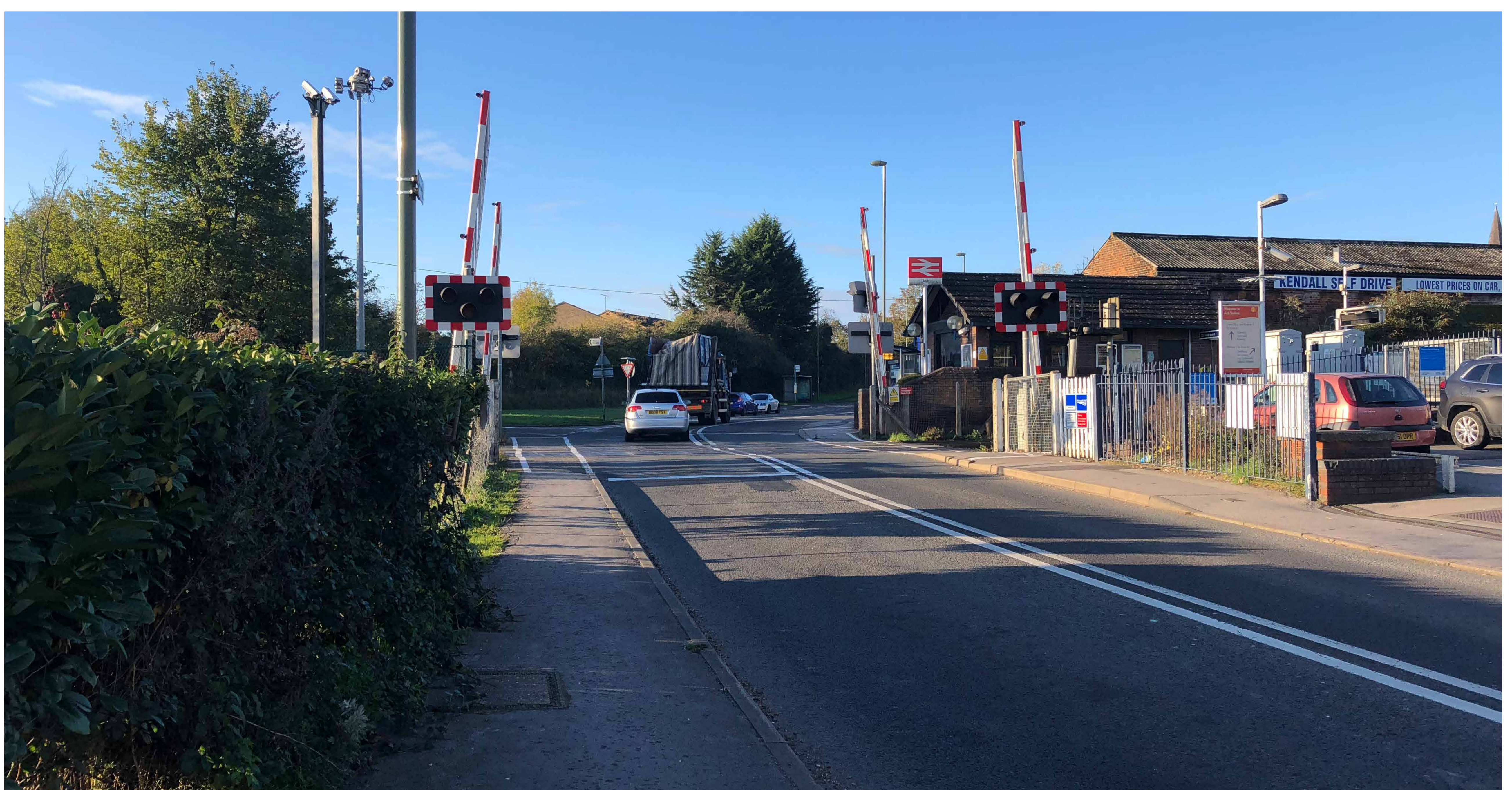
Ash Level Crossing (looking south west)
