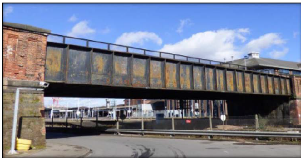
Figure 6: : Farnham Road Bridge and access road to Farnham Road car park
