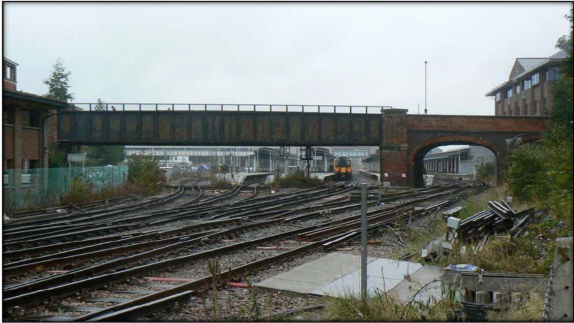
Figure 5: Farnham Road Bridge
