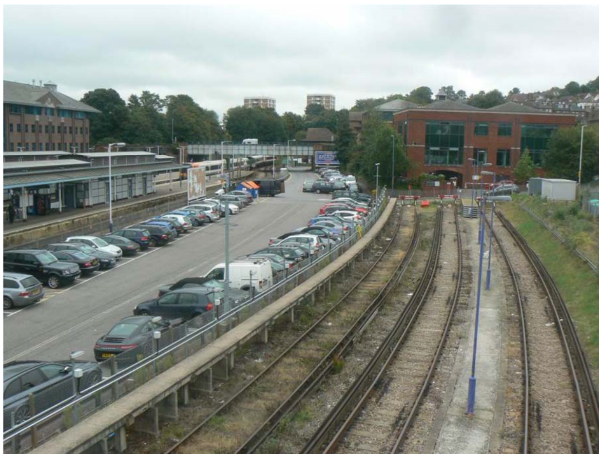
Figure 4: west side sidings
