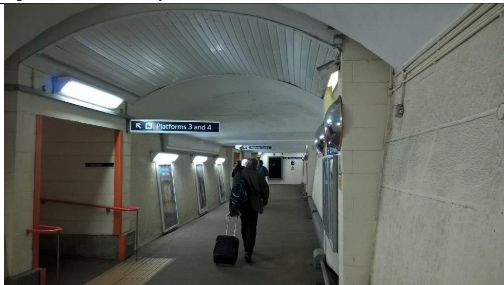
Figure 6 – View of subway
