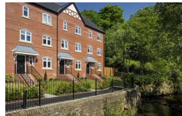
Strong residential frontage along the river
