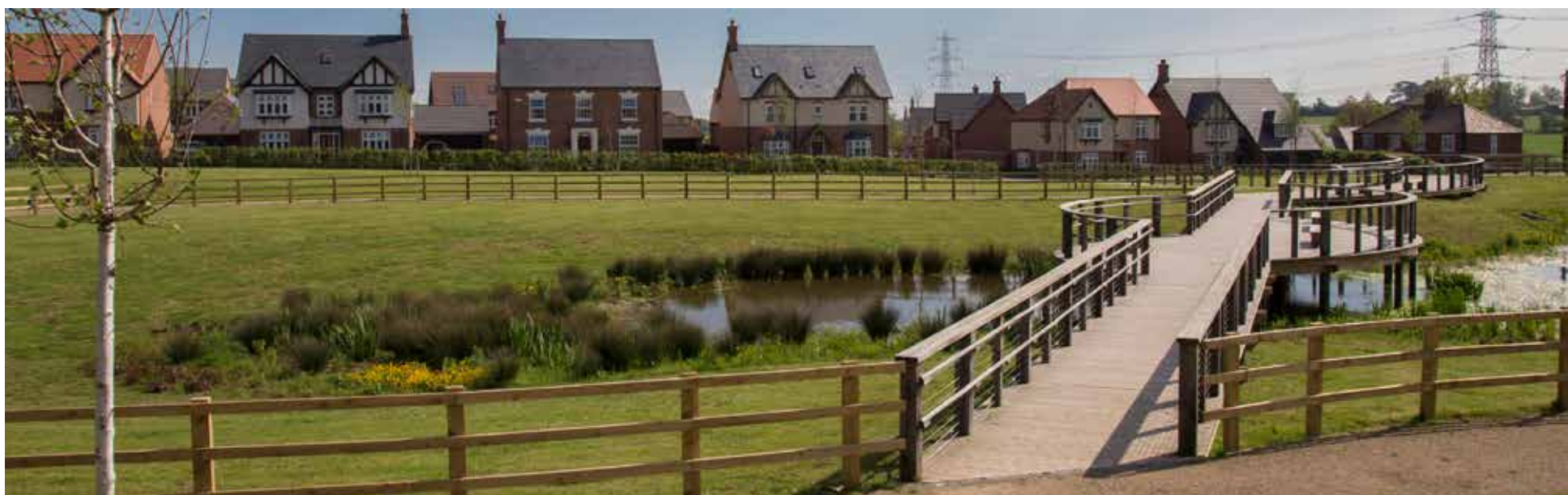
Dwellings overlooking a green landscape with integrated swales
