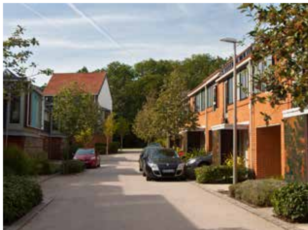
Shared surface tertiary street
