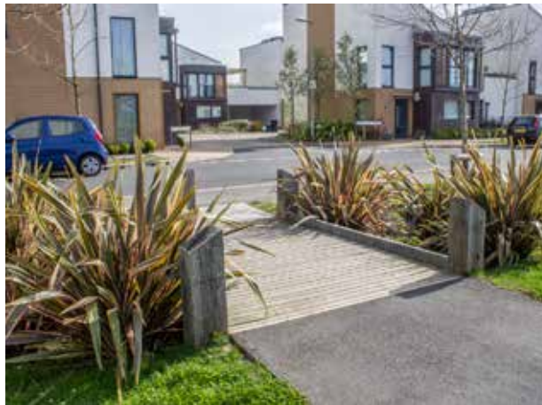
Swales integrated into the streetscape to provide linear green corridors.
