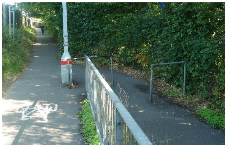
Inappropriate barriers on path alongside A3, not conforming to Equality Act (common)
