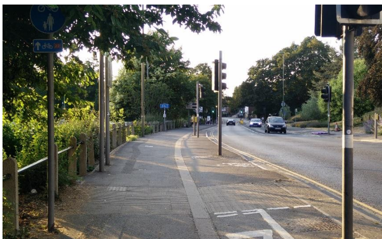
Signal posts compromising cycle track along Shalford Road
