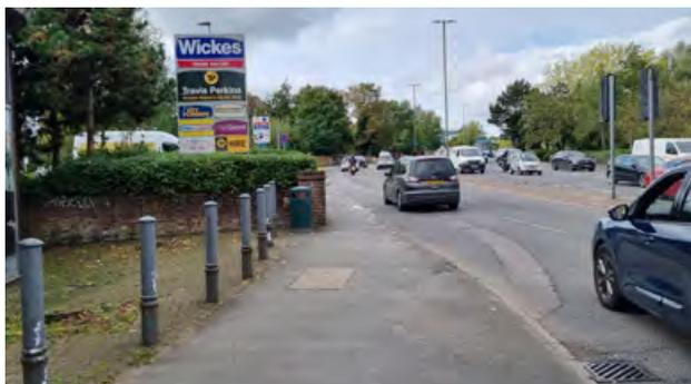
Figure 65. Existing shared use paths on the A25 have inconsistent width and at locations are very narrow. Improvements to the facilities are required to enhance the connectivity of the network.
