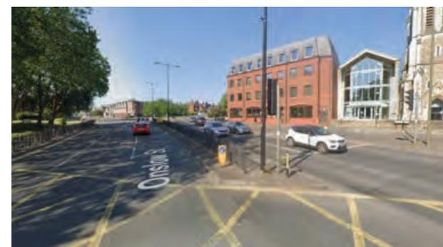
Figure 58. Onslow Street: dual carriageway with high traffic flows. Existing footways have guardrail. Opportunity to widen the footways to accommodate shared use path to provide access to the town centre. Source: Google Street View.
