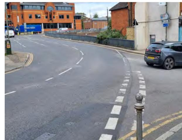
Figure 54. Park Street/ High Street junction: wide bellmouth allows for high turning speeds and limits the space for pedestrians and cyclists.
