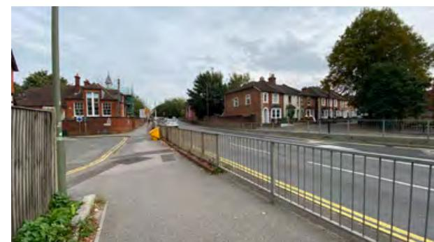
Figure 57. Level difference between Artillery Terrace and York Road will be required to be resolved following the implementation of the new crossing.
