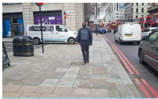
Raised Table (Side Road Entry Treatment) Reinforces the Highway Code 2022 update by enhancing priority for people walking and wheeling and making the side road crossing easier and more convenient by maintaining the continuity of the corridor at footway level. It indicates pedestrian activity, encourages lower traffic speeds, and more driver attention. Variations also referred to as a continuous footway, blended crossing or Copenhagen crossing, as shown above.
