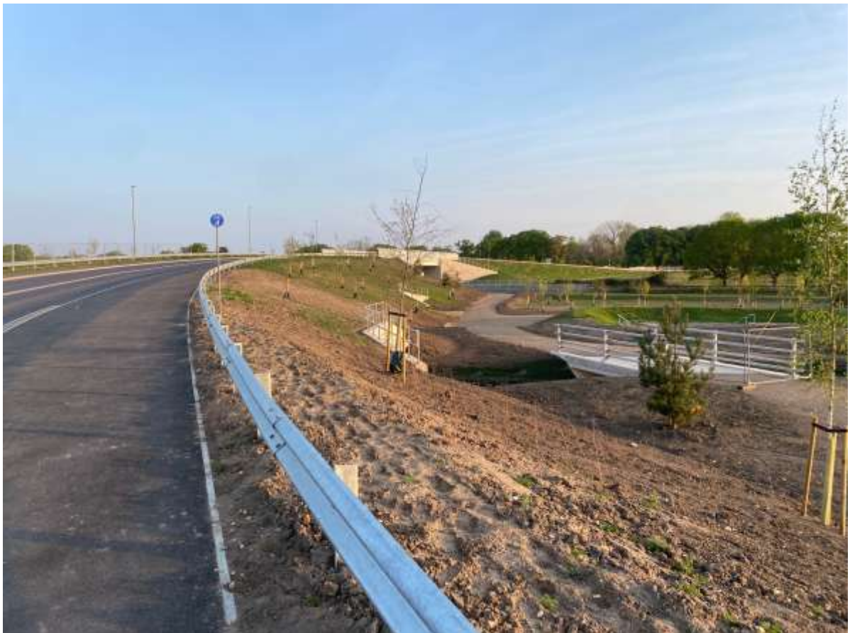
Figure 2 New Ash Bridge, removing the need of level crossing for vehicles
