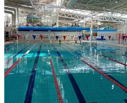
Photo: Pool covers stored on their roller systems [photo courtesy of Freedom Leisure].
