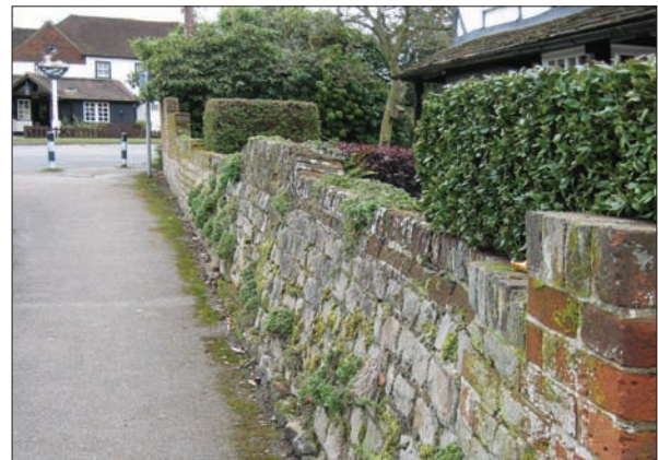
Walls at front of Hatchers on the Green
