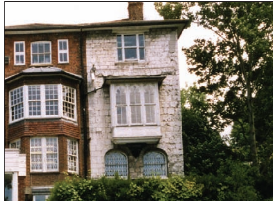
Clunch is used on the rear elevation of this building facing Millmead
