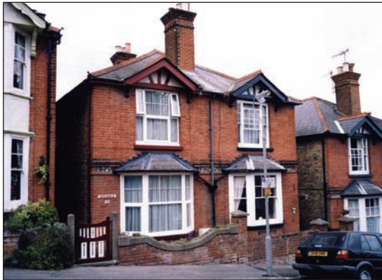
Slate roofs in Brodie Road
