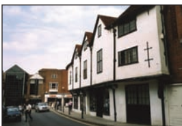
Timber framed buildings in Quarry Street
