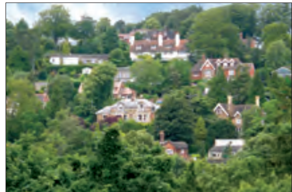
hillside housing within spacious landscape grounds
