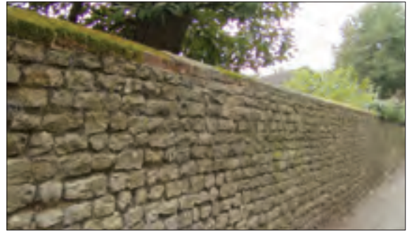
Bargate stone wall in Portsmouth Road
