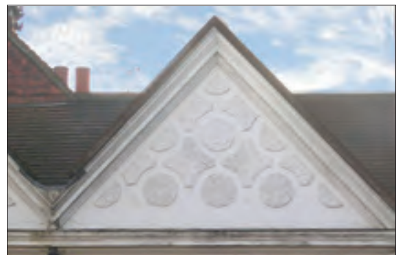
gable of 50 Portsmouth Road
