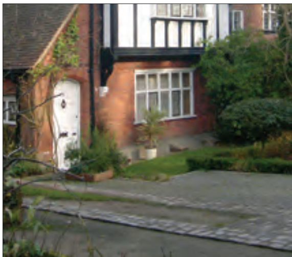
encroachment for parking
