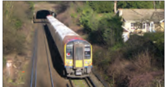
railway cutting and tunnel
