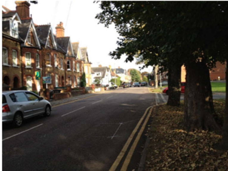
FIGURE 4.5 YORK ROAD LACK OF SIGNS
